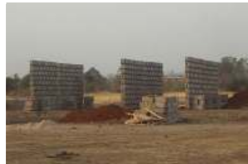
3 new classrooms for the Lighthouse
