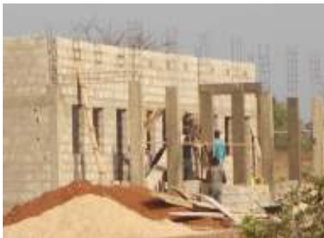
New PTI dorms under construction
